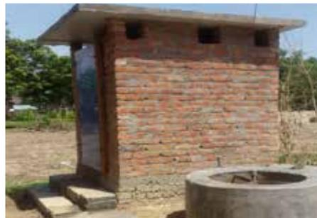
Figure 4: Toilet attached to Biogas plant in Kailali
